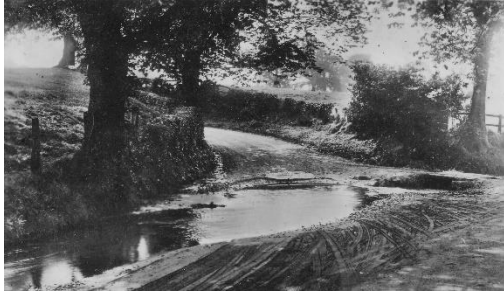
Fanshawe Brook before the culvert was built in 1938 (original kindly loaned by Jess Ford)
