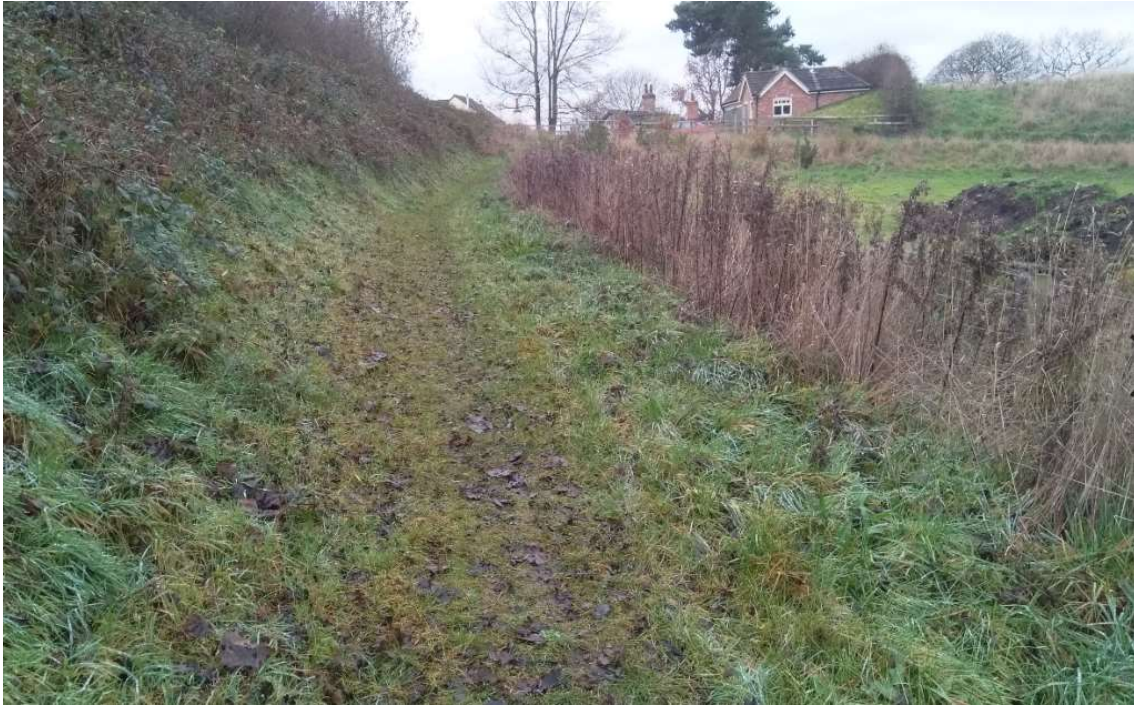
Path from the gateway towards Henbury Moss. It is in good condition. This is what we inspected a couple of years ago.
